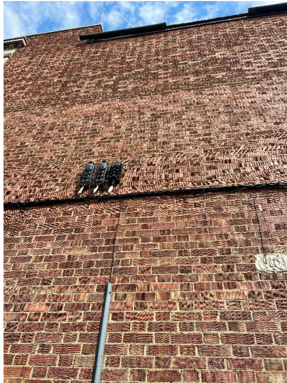
Photo 13 – General view of the side elevation brickwork
