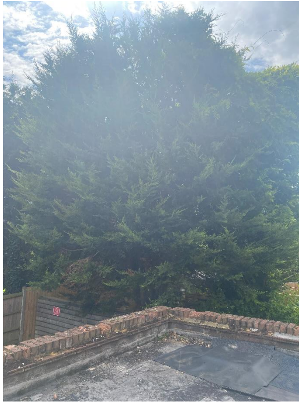
Photo 23 – General view of the tree looking rom the extension roof
