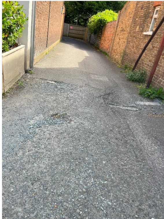
Photo 8 – General view of the side access to the rear of property
