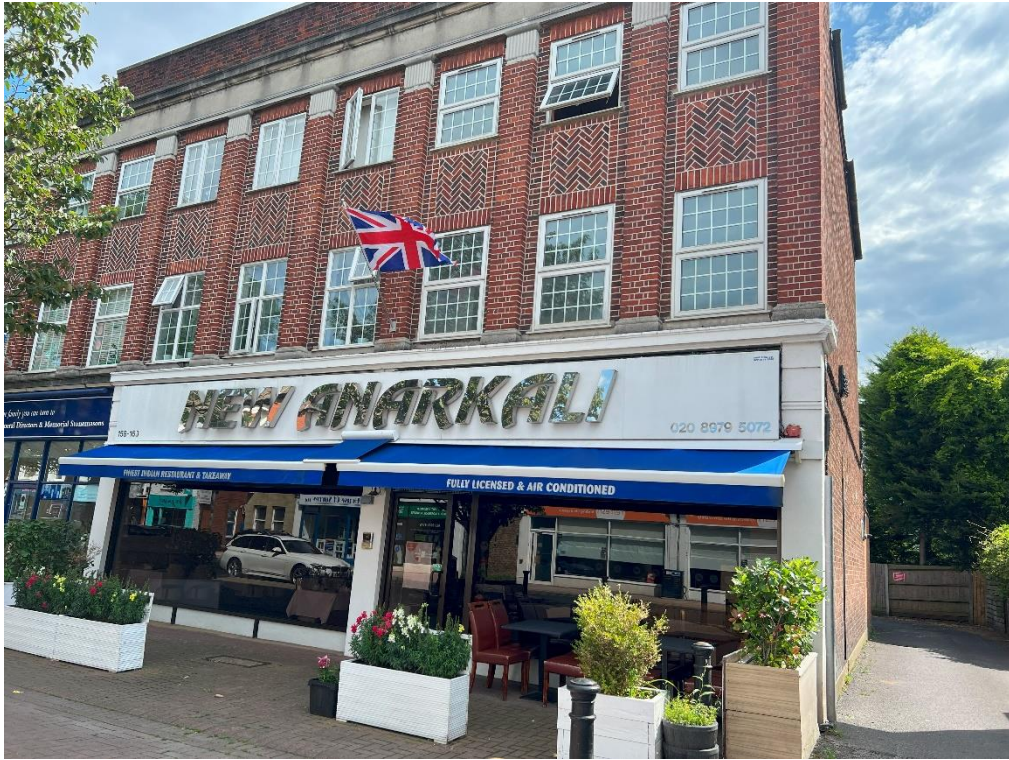
Photo 1 – General view of the front elevation
