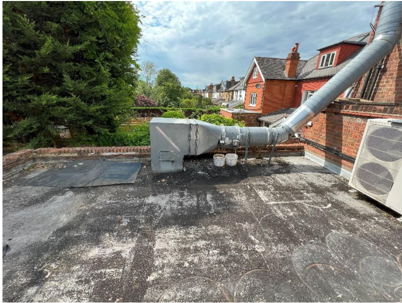
Photo 5 – Rear Extension roof
