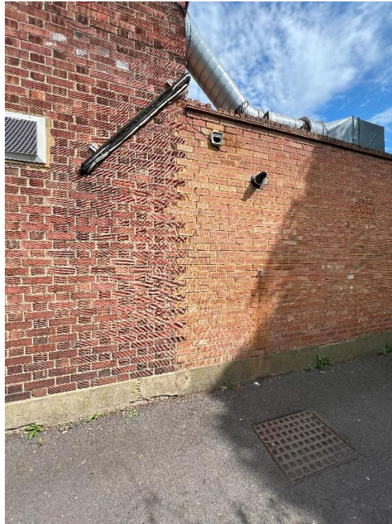
Photo 9 – Junction of original building and rear extension
